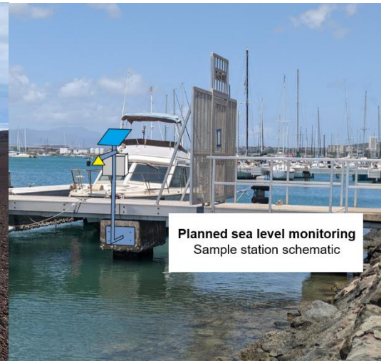
Figure 2: Each new tide gauge station will include a radar sensor to measure water level, solar power, and satellite telemetry (yellow, blue, and gray shapes, respectively), as well as long-term leveling controls.
