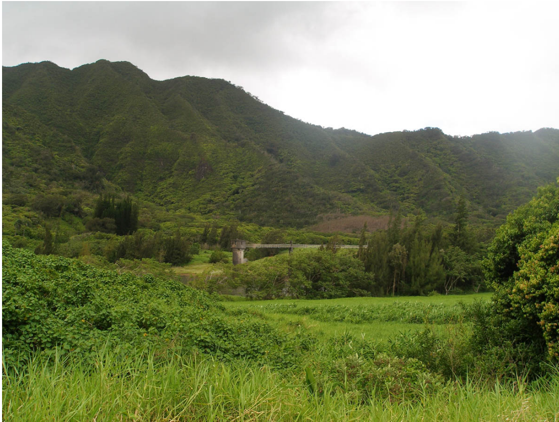
Figure 11. The Nu'uaniu reservoir and watershed area on the Island of O'ahu. (Source: Honolulu Board of Water Supply)
