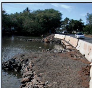
The damaged park and eroded beach road next to the Humpback Whale Sanctuary in Kihei, Maui, shows how potentially vulnerable Maui is to storms and climate phenomena. After an abnormally rainy La Niña winter season, beaches and shoreline infrastructure were already affected when surge from the Japan earthquake caused additional damage. (Photo credits: Dr. Victoria Keener.)
