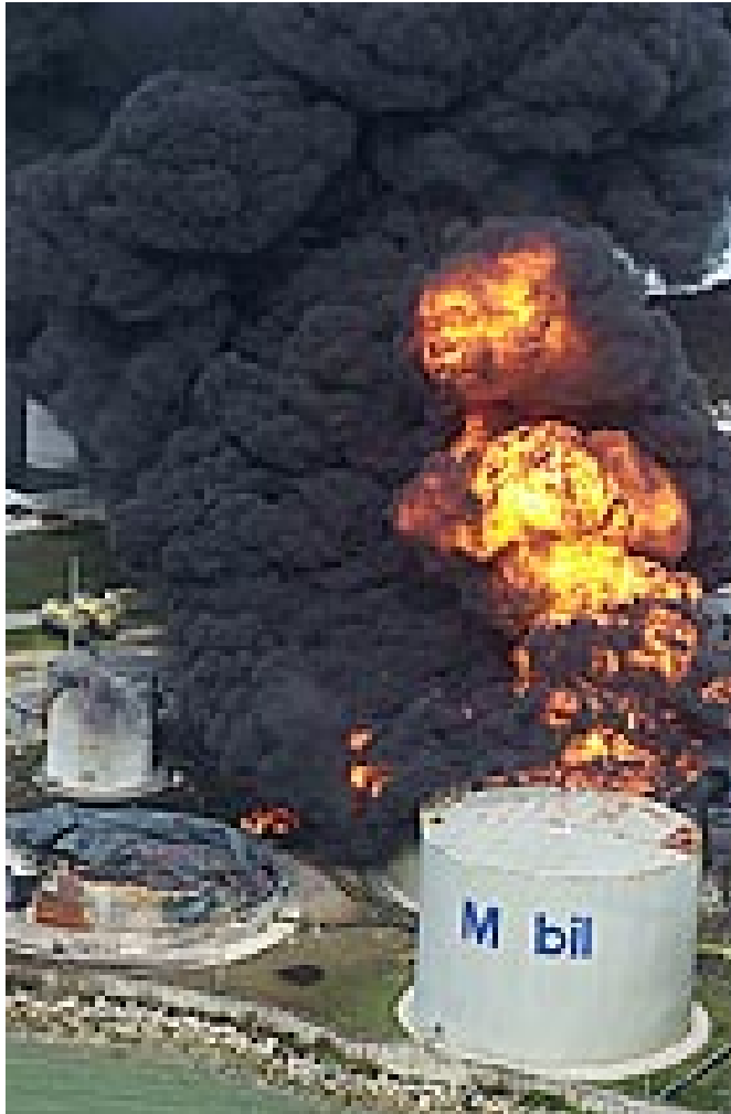
Burning fuel tanks after the passage of Supertyphoon Pongsona (photo from Guam Pacific Daily News Ron Soliman)
